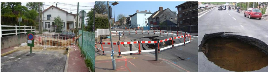
Figure 3. Examples of sinkholes in the principal European capitals a) Paris, b) London and c) Rome (Parise, 2012, Edmonds, 2018, 10 Leparmentier, 2013).
