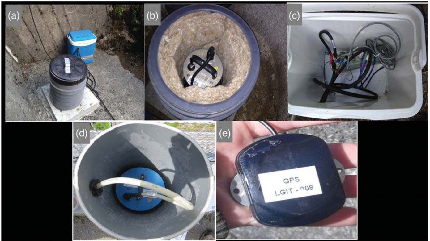
Figure 3. Station details. (a) Final installation of a station along the dam–rock interface. (b) The gray plastic cylinder sealed within the concrete slab contains the CMG40T sensor surrounded by a thermal isolation wool, and (c) the blue plastic device contains the Nanometrics Taurus digitizer and its cables. (d) The Lennartz-3D-5s sensors installed on the crest of the dam use smaller plastic cylinders and no thermal isolation. (e) A Global Positioning System (GPS) receiver is added to each station for time synchronization.
