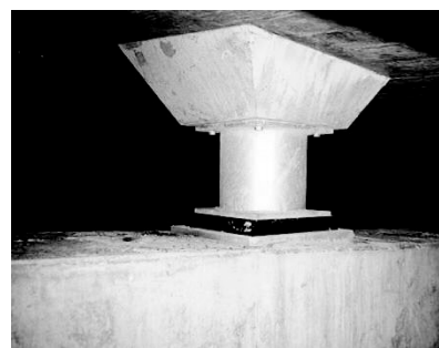
Fig. 5 – Fuse - support of the slab - Tonello IC - dossier IVOR.
