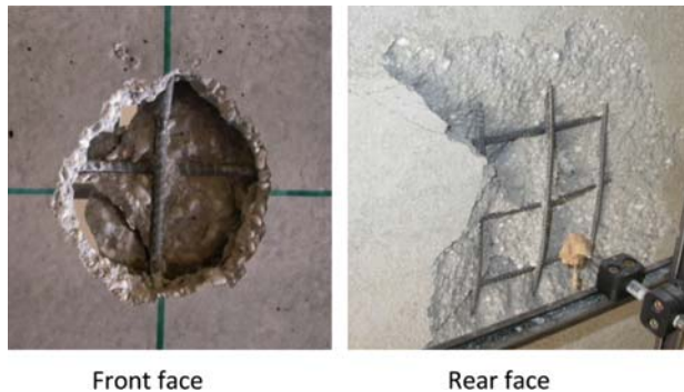
Figure 6. Damage on the reinforced concrete slab after test no. 2, V_0 = 70.2 m/s.
